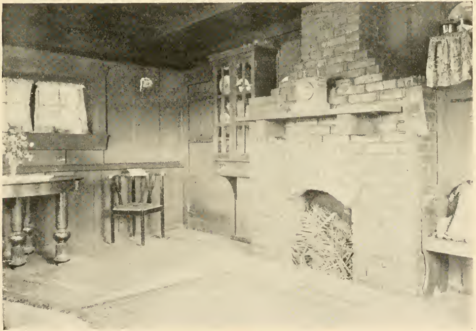
The Brick Deeply Revealed by the Pointing
